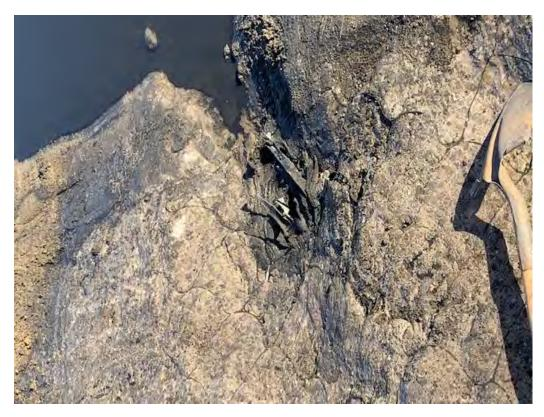
Figure 1 - Visual Identification of Primary Liner Damage – Shovel on the Right for Scale
