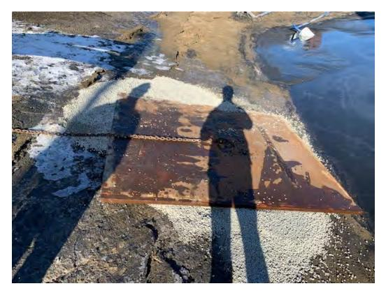
Figure 2 - Temporary AquaBlok Backfill and Steel Plate Placement
